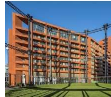
Kings Cross Central – design & engineering across 15 sites
